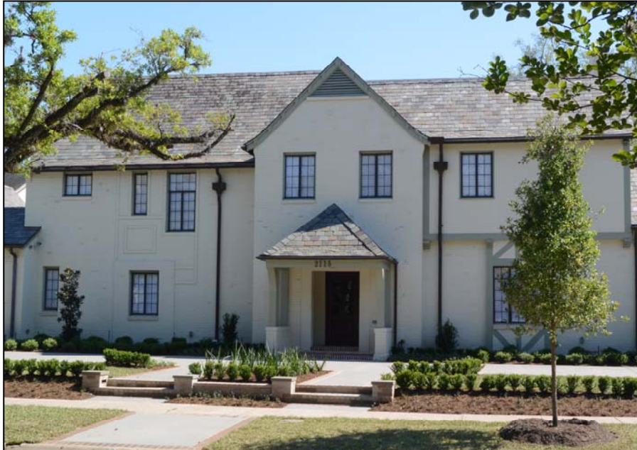
2115 Glen Haven Blvd..
