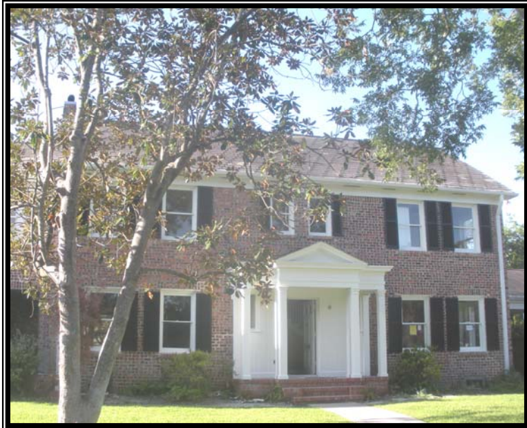
2305 Glen Haven Blvd. is undergoing renovation.
